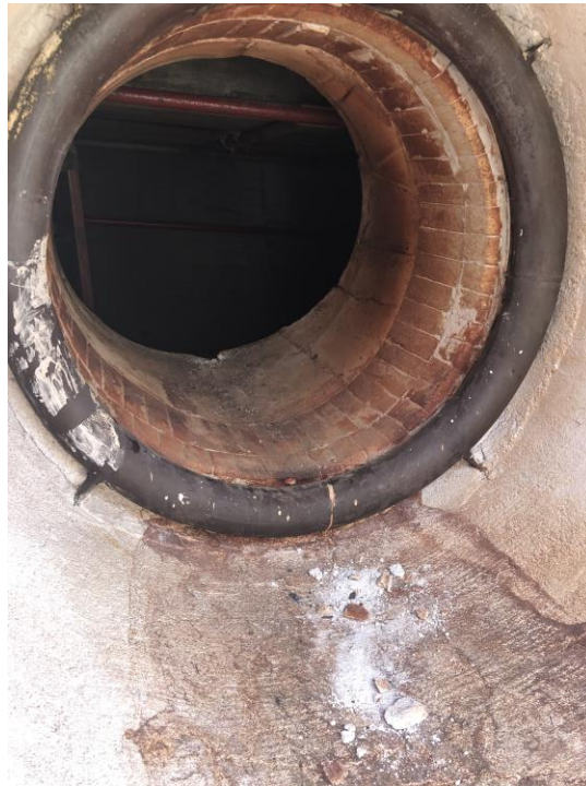
Tangential ring type burner
